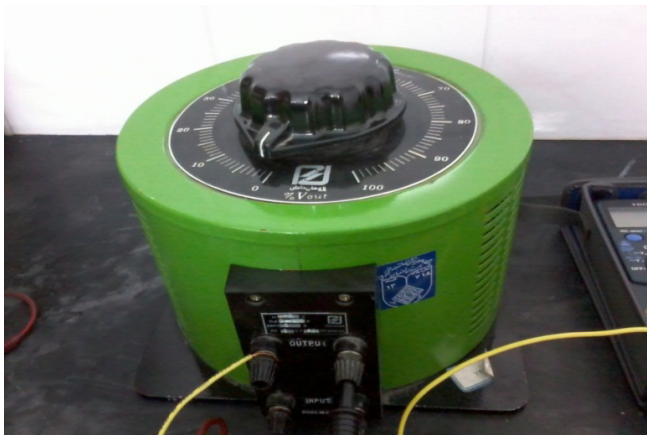
Figure 1: The Autotransformer.
